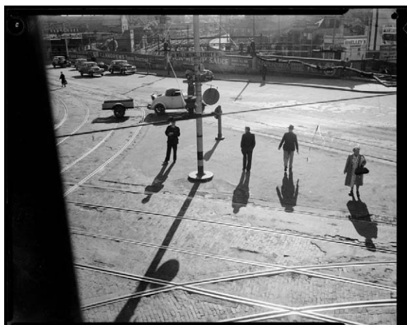
Newtown Bridge, scene of a fatal accident. Police Photographer Nixon, 1950.
