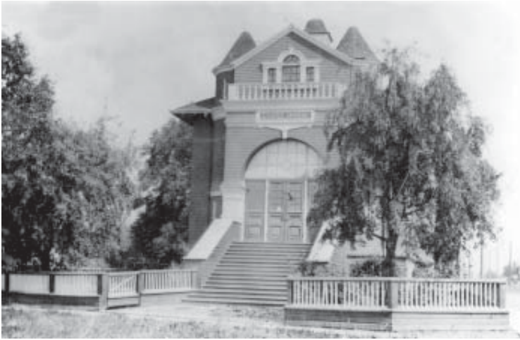
Figure 4: Chilliwack Courthouse, designed by F M Rattenbury, opened in 1894; photograph c1900. Reproduced by permission of British Columbia Archives.
